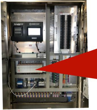
The ISOFuel Modules allows the user the ability to configure a fuel system to easily function with any ATG manufacturer and control any STP, whether they are using contactors, SC controllers or VFC drives.
